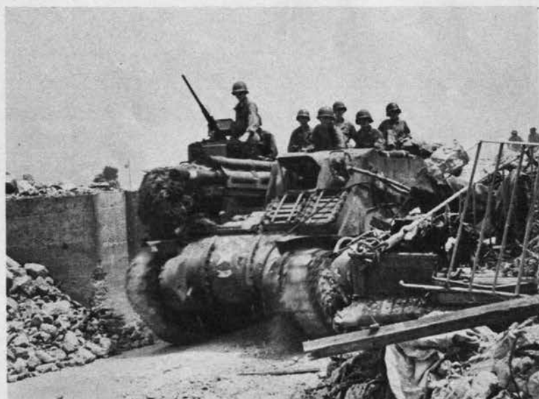
Grim-looking vehicle is U. S. M-7, the Priest, an SP 105-mm. howitzer on a medium tank chassis. The hull is built high in front with sloping bow and distinctive pulpit-like AA ring mount. The M-7 has no turret.
